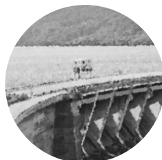
Power Generation Kashimbila Dam
